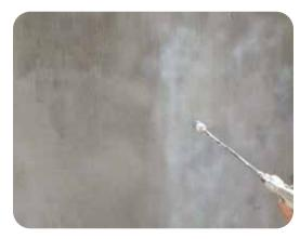
STUCCO CONDITIONER is an efflorescence preventative blocker which may also be used as a penetrating hardener and pH neutralizer. May also be used as a primer for acrylic and elastomeric finishes and other synthetic stucco. Stucco Conditioner will harden and restore soft stucco and other cementitious materials.
